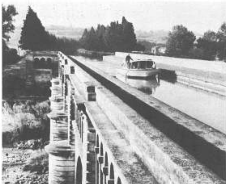
The Canal du Midi crosses a river in Southern France
