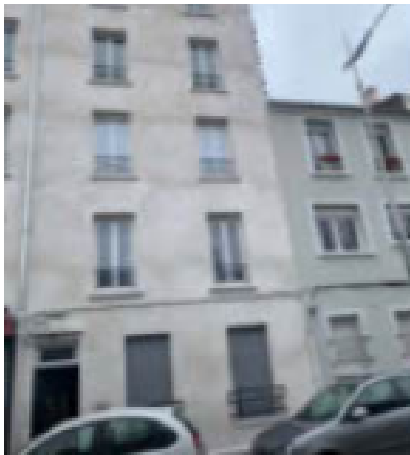
Building Entry /Entrée du batiment
